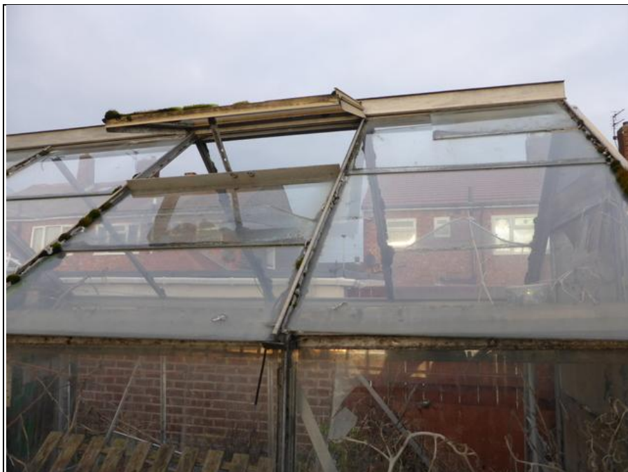
Skylight still functions.
